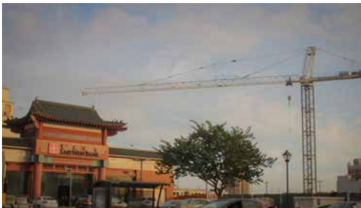
Construction of Blossom Plaza at Chinatown's Entrance (Photo by Cameron Quon)
